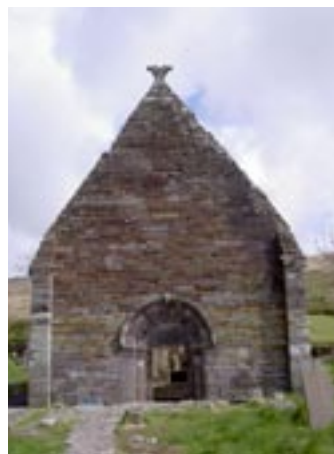
Fig. 1 The Romanesque Church at Kilmalkedar, West wall.
